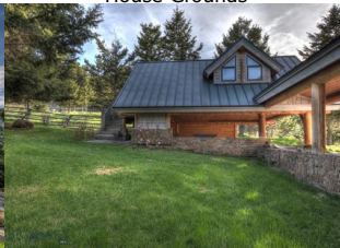
House carport with extra room above.
