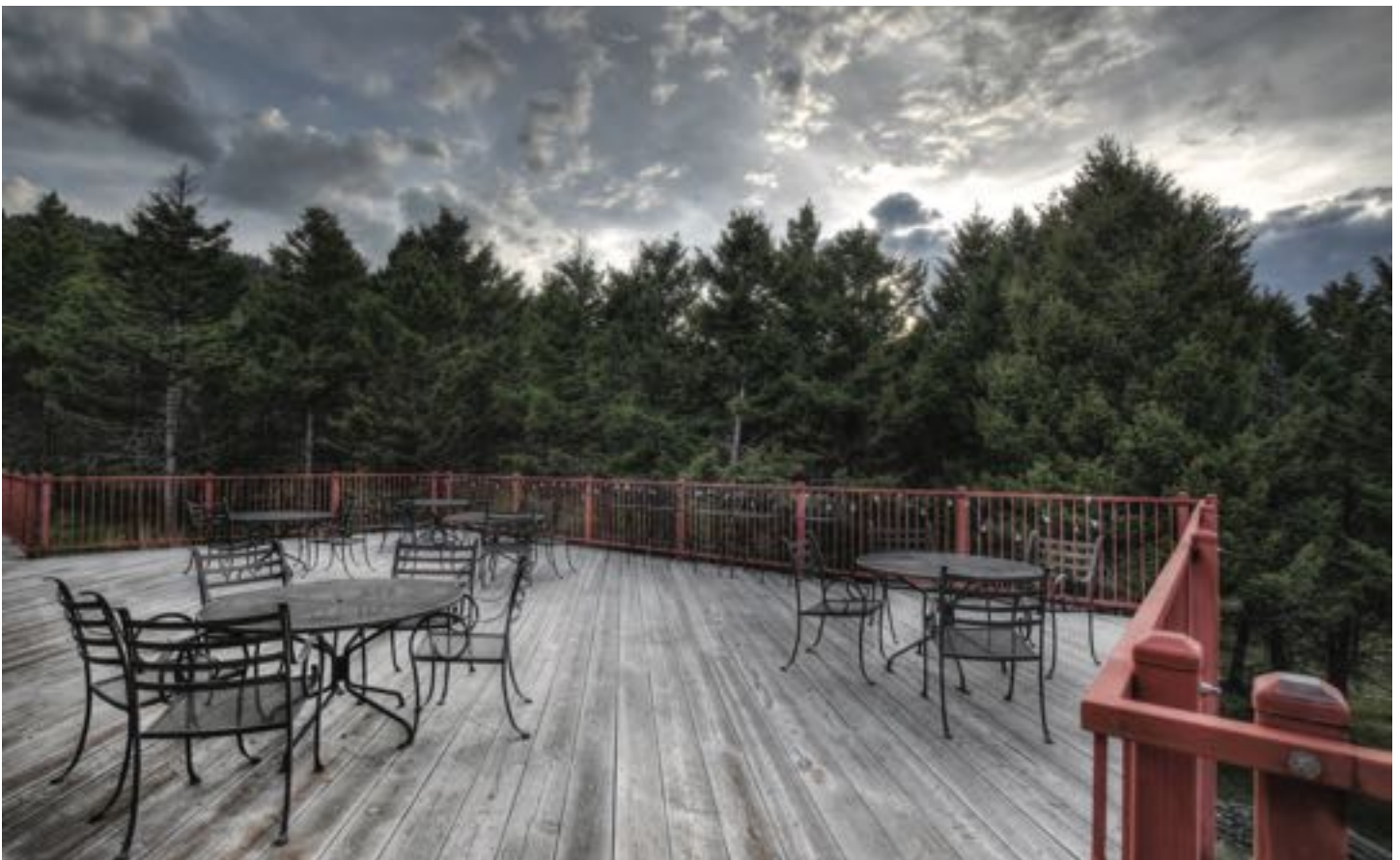
Second floor surrounding deck made of solid Cyprus with powder coated steel supports and railings
