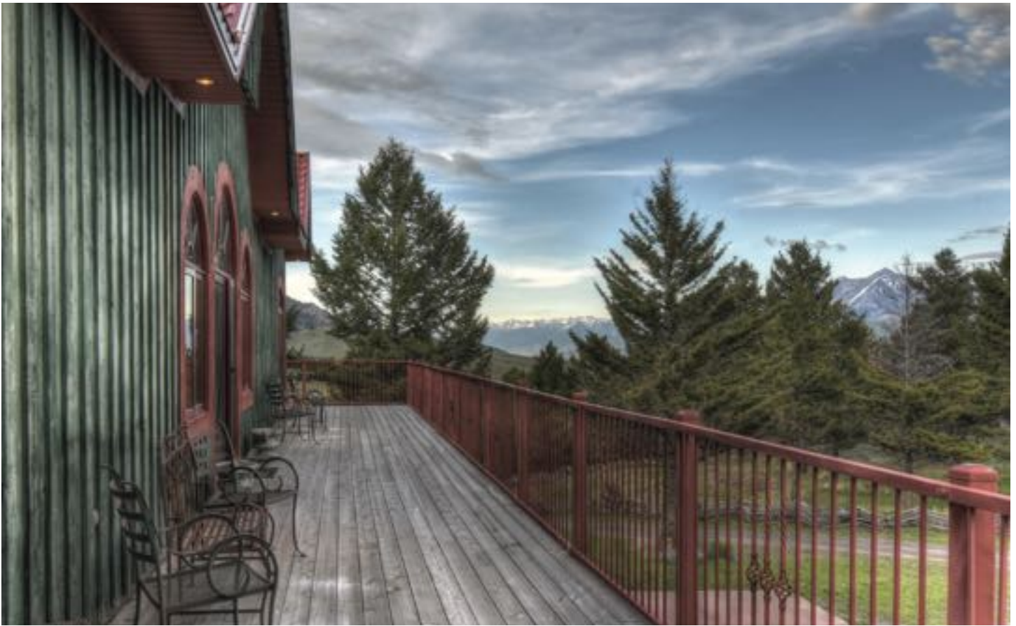
Second floor surrounding deck made of solid Cyprus with powder coated steel supports and railings
