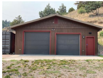
the 960sq. ft shop/ garage heated
